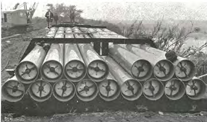
The 16 eight-inch diameter tubes, complete with end stoppers, assembled in the lifting cradle on the river bank.
