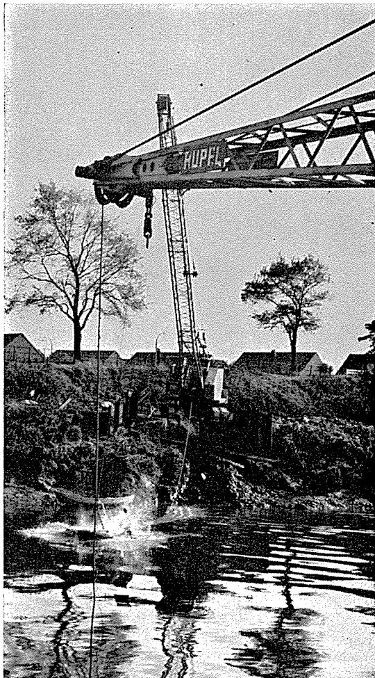
Two cranes operating drag-lines work from opposite banks excavating the deep trench in the river bed.
